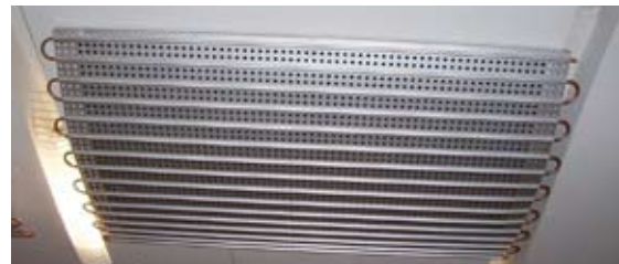
Figure 2. The final panel design with a perforated acoustic backing panel
