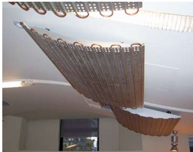
Figure 7. Version 3 – three versions developed at different levels of curvature, middle one is the final system
