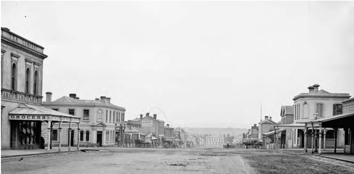
Figure 23 Looking east along Faraday Street, c. 1870s, with Lygon Street crossing in the foreground. King & Godfree's premises is at left, then a tea merchants' shop Source: American & Australasian Photographic Company, FL1250690, Mitchell Library, State Library of New South Wales
