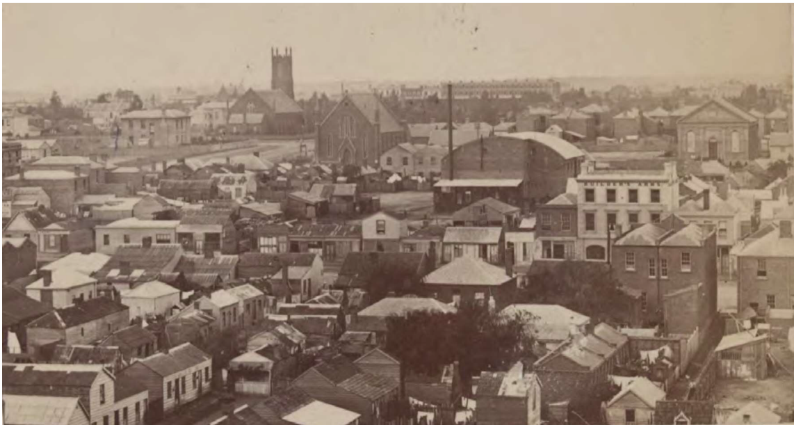
Figure 2 View of Carlton between Queensberry and Victoria streets in 1870, looking east past Cardigan Street towards Carlton Gardens, 1870 Source: Charles Nettleton, photographer, H96.160/1433, State Library of Victoria
