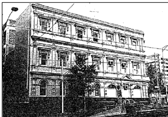
Figure 7 Image from the 1985 CAD study showing altered ground level openings since restored.
