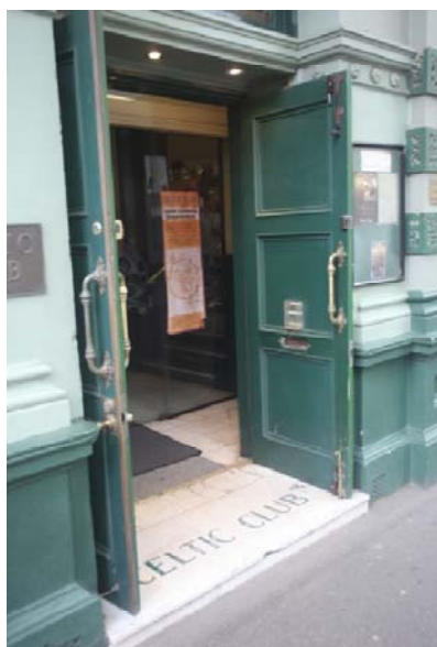
Figure 14 Queen Street entry point
