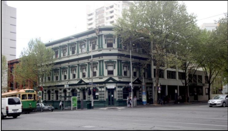
Figure 1 former West Bourke Club Hotel 2010
