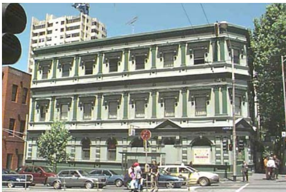
Figure 8 Image from the 2002 review showing altered ground level openings
