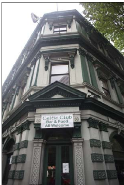
Figure 15 rich detailing of the facade
