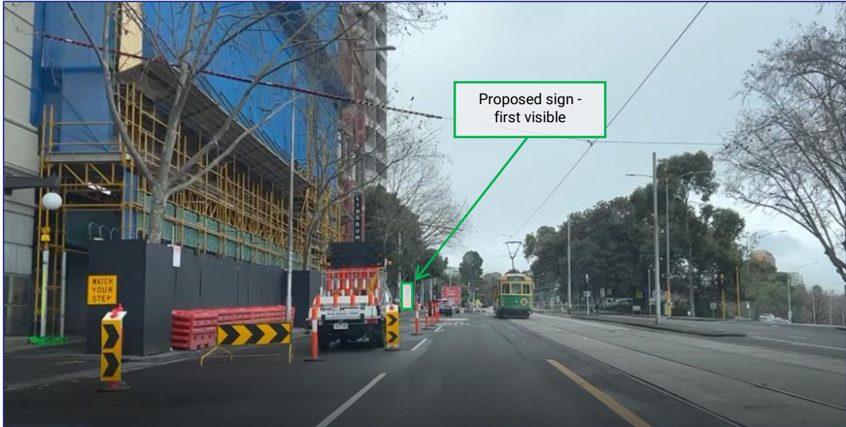
Figure 32: 1 Spring Street - Sign first visible on eastbound approach
